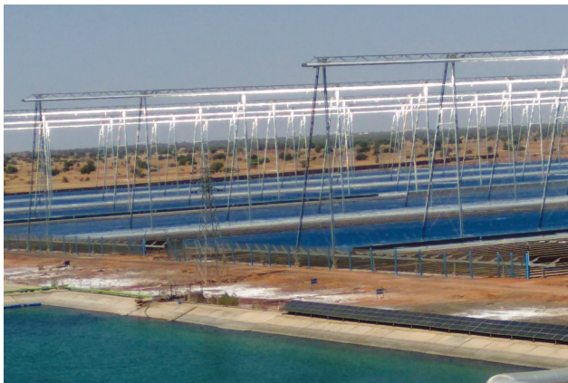
Figure 2: Reliance CLFR plant during operation at Dhursar
